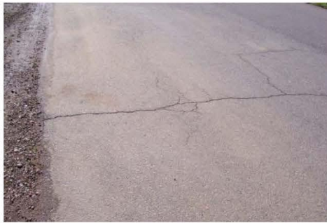
Transverse Crack
