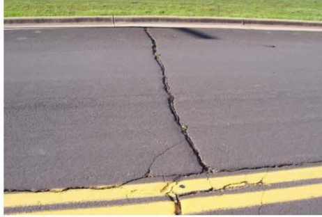
Transverse Crack
